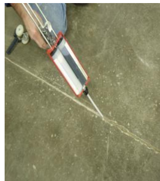
Crack Repair
